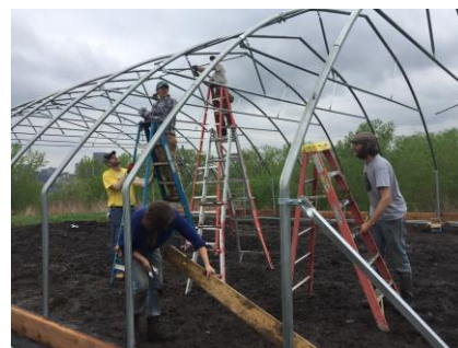
Nick Krueger (yellow shirt) helps a team from Urban Roots assemble the frame for a hoop house, which can be used to extend the growing season for produce. The final part of the project involves wrapping the frame with a plastic cover.
