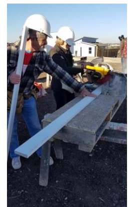
Linda Bishop (on right) using a miter saw to cut exterior molding.
